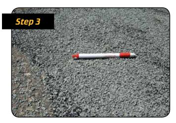
A fine aggregate cover material is applied over the sealant. The cover material has the added benefit of improving the ride of the surface.
