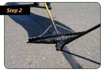
FLEX-PATCH is applied through a wand and then hand squeegeed to insure proper coverage. A sufficient amount of sealant is applied to flood the entire distressed area and provide an 1/8" base to hold the final cover material.
