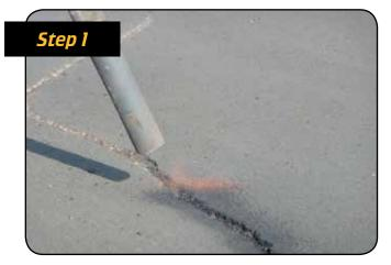
Fahrner crews clean and dry the area using air compressors with a minimum of 100 psi and heat lances with a minimum temperature of 2200 degrees. Sealant will not adhere to dirty or wet surfaces.
